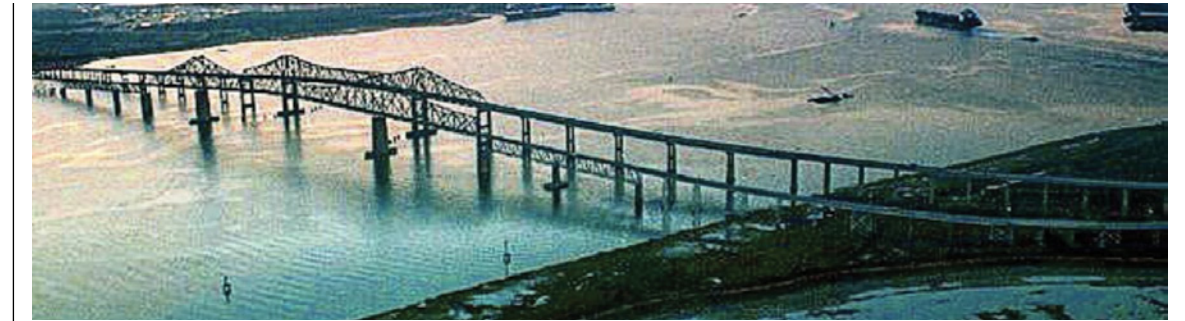
GRACE MEMORIAL AND SILAS PEARMAN BRIDGES | PHOTO BY CHARLESTON CORPS
