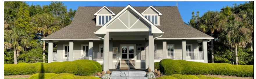
Seabrook Island Town Hall
