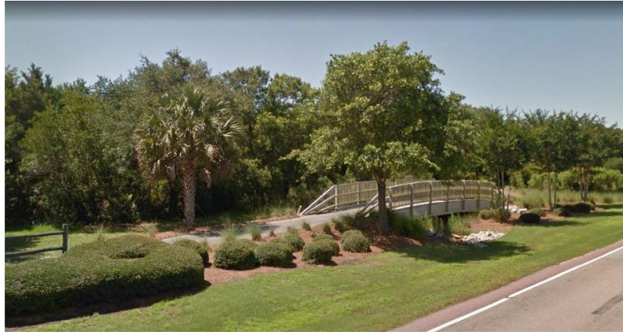
Shared Use Path, Seabrook Island Road
