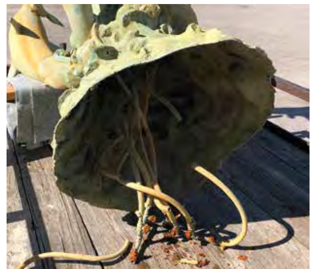
Old pipes rusted - not in working condition
